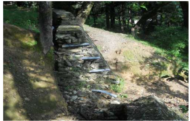
Figure 15 Provision of weepholes in normal construction and ill performance due to poor maintenance
