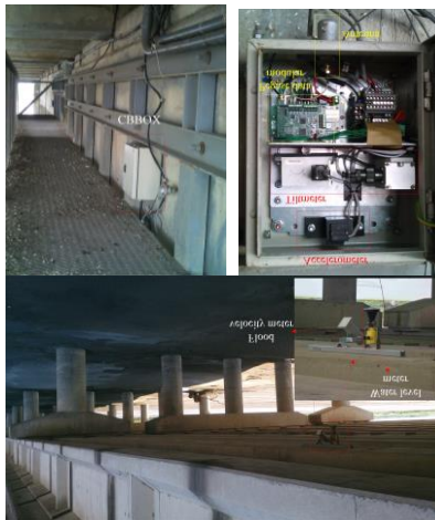
Figure 14 Installation of the intelligent performance monitoring system on Xibin Bridge
