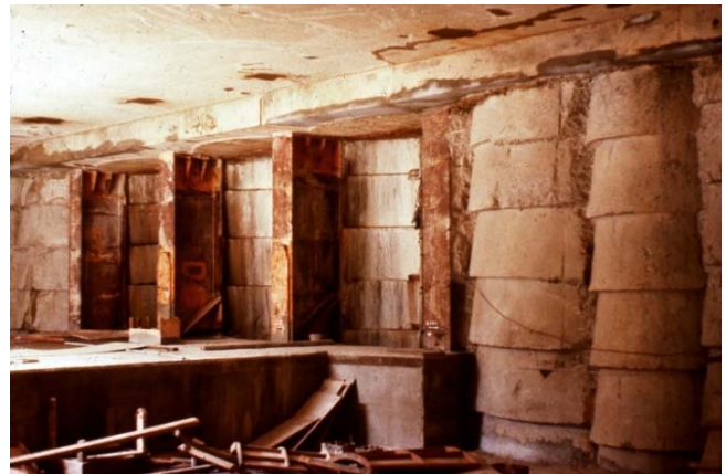
Figure 1 Hand dug caisson walls
