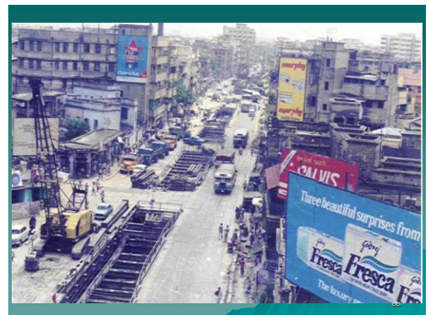
Figure 8 Cut and cover construction through Chittaranjan Avenue
