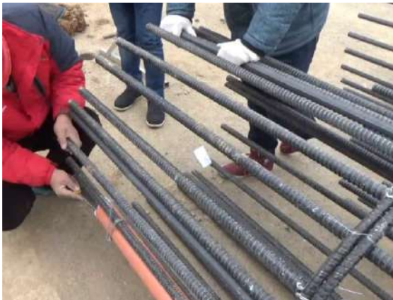
Figure 8 PVC Tube on GFRP Cage
