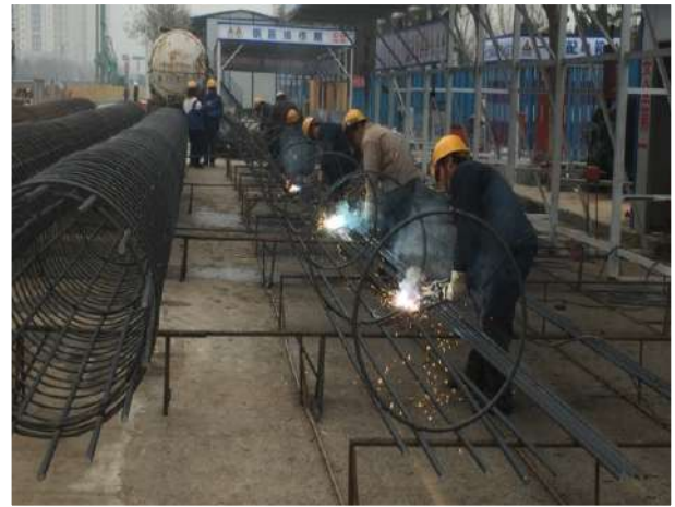
Figure 7 Assembled Steel Cage of Pile
