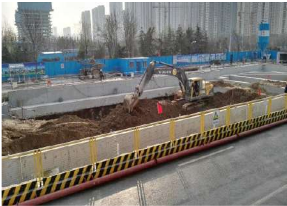
Figure 12 Excavation after First Concrete Support was installed
