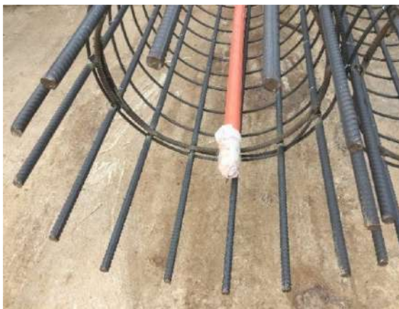
Figure 9 PVC Tube on Steel Cage
