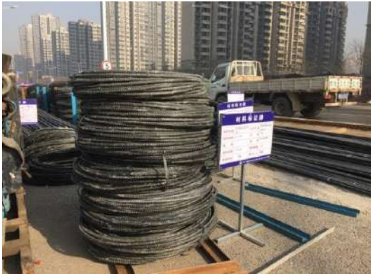
Figure 4 GFRP Stirrups of Piles
