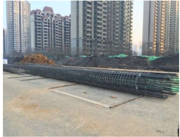
Figure 6 Assembled GFRP Cage of Piles
