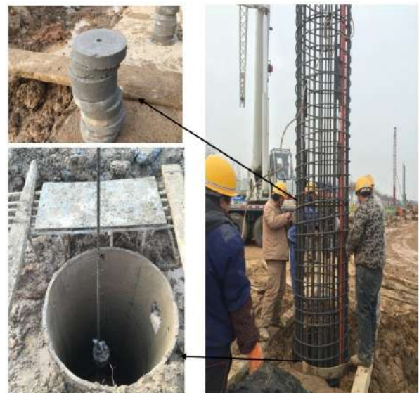
Figure 11 Installation of Steel Reinforced Concrete Pile
