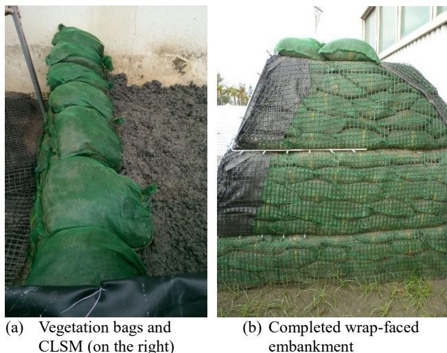
Figure 9 Construction of wrap-faced reinforced embankment using pervious-CLSM
