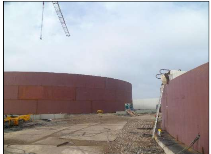
Figure 2 Fuel tanks under construction at Ostend (Belgium) – fall of 2012.
