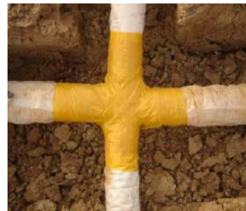
(b) Connections of horizontal and longitudinal main pipe
