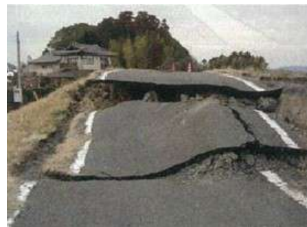
(a) River dyke failure
