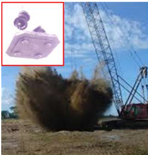
Figure 11 Moment when Pounder Hits the Ground
