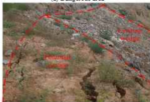
(b) Cracks on the third-level platform
