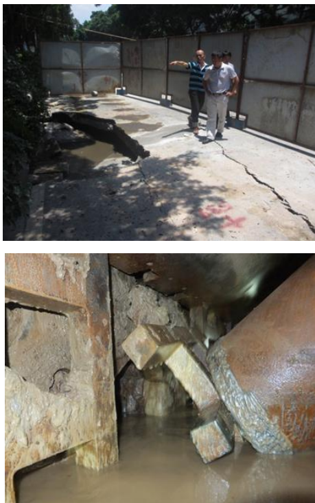
Figure 7 Grille deformation of shield
