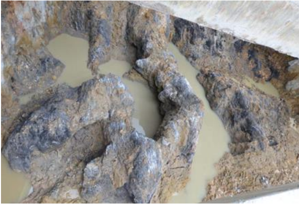
Figure 2 Groundwater condition in limestone section of north extension section of Guangzhou Metro Line 8
