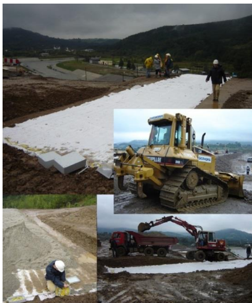
Figure 3 Installation of a GOF-based non-woven geotextile in a gravity dam in Swina Poremba, Poland
