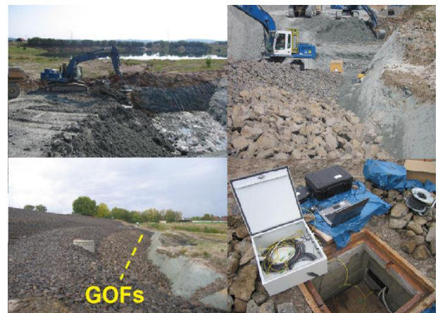
Figure 6 Installation of GOF-based geosynthetics at an abandoned opencast pit at a depth of 7 m in Zimmersrode, Germany
