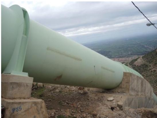
Figure 3 Water pipeline in steep terrain with more than 500 individual segments
