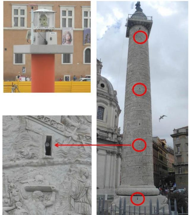
Figure 2 Monitoring of the historic Trajan's column with a robotic total station and prism targets
