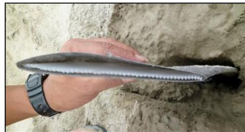
Photo 4 Installed prefabricated vertical drain
