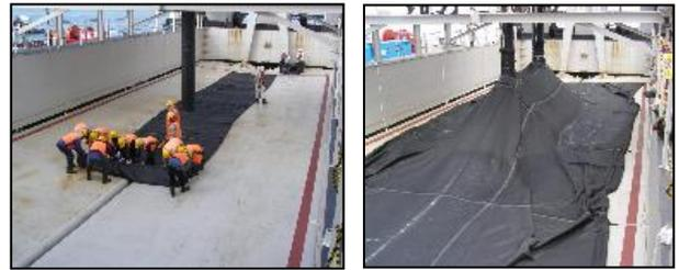
(1) Laying of empty tube (2) Filling CMS into tube
