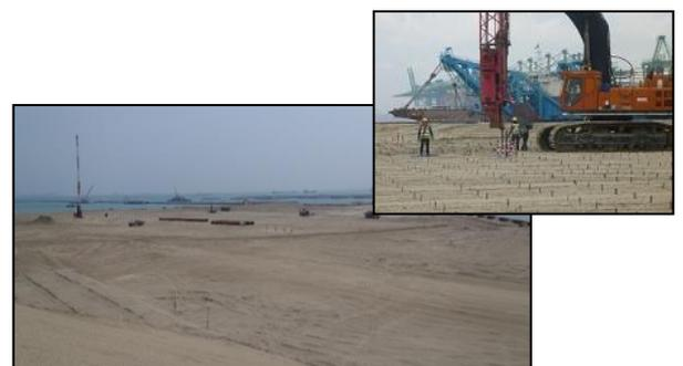
Photo 3 Reclamation of sand fill and PVD installation
