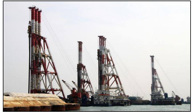
Figure 19 Sand compaction pile (SCP) application
