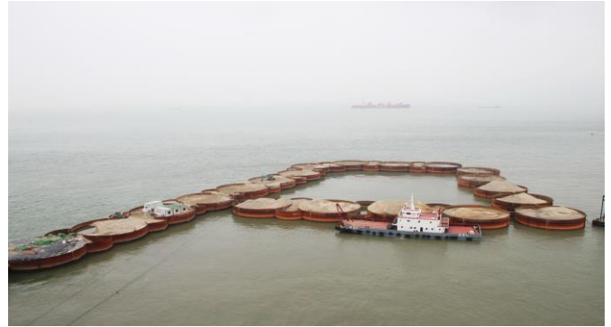
Figure 7 West artificial island smaller island reclamation
