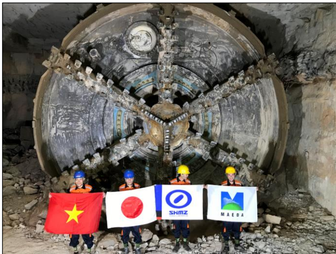
Figure 16 Exposed TBM after arrived in Opera House Station B4F
