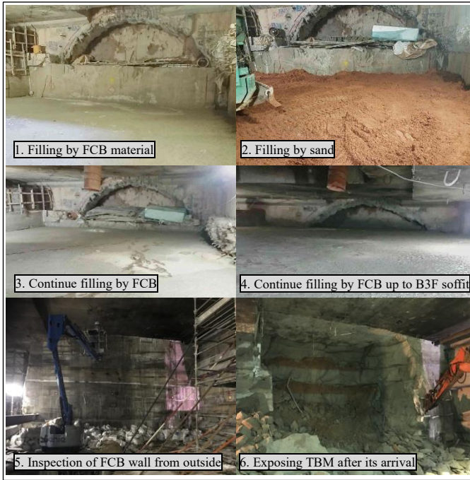
Figure 15 Construction of FCB and sand backfilling used to receive TBM at Opera House Station B4F (number indicates construction order)
