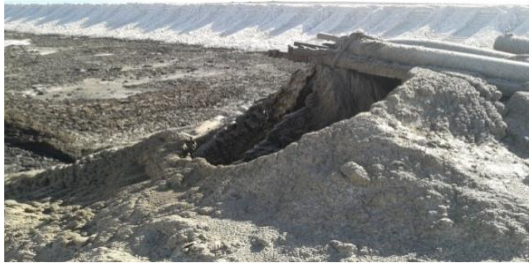
Figure 1 Pipes reversing Phosphogypsum sludge via wet process – Sfax Unit
