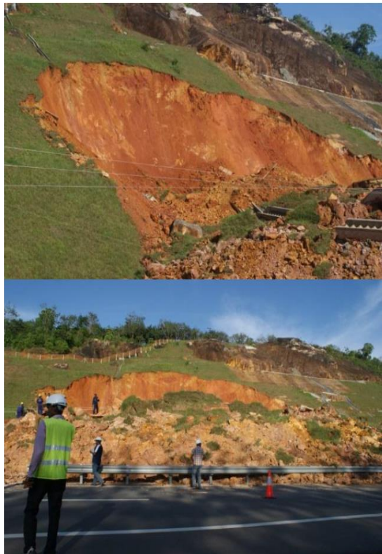
Figure 1 Failed slope of Southern Transport Development Project (STDP) at Welipenna
