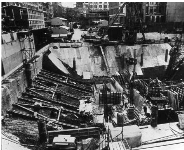
Figure 2 Photograph (taken August 1963) showing basement construction of Britannic House with strutting: observation casing and access scaffolding visible on left (Cole and Burland, 1972).
