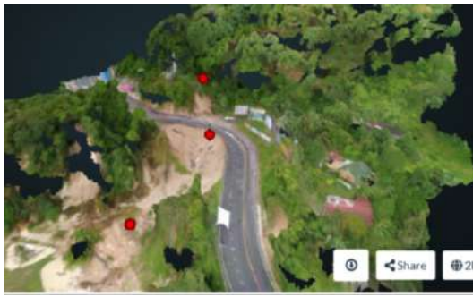
Figure 8 3D-model of the slope based on UAV survey
