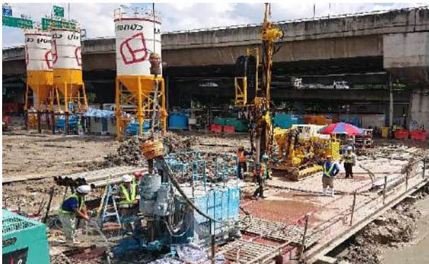
Photo 7 Construction in Thailand
