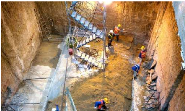
Figure 19 Final excavation base at a depth of 32.5 m for TBM shaft
