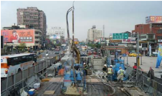
Photo 6 Construction in Taipei, Taiwan
