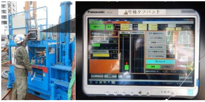
Photo 4 Construction monitoring device
