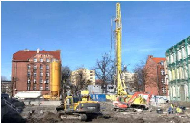
Photo 5 Construction in Europe
