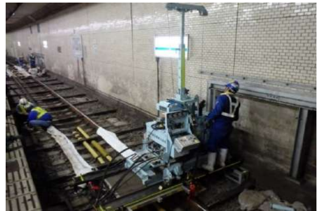
Photo 2 Construction inside subway station with a small machine
