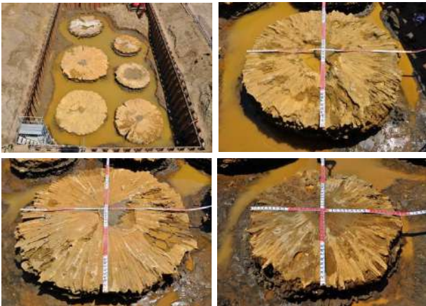
Photo 1 Excavated jet grouting (Shinsaka et al., 2013)
