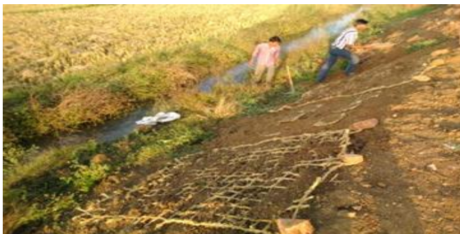
Figure 4 PSGs, being laid on Canal slope
