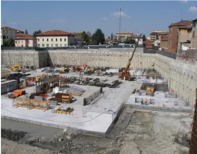
Figure 13 a), b) Excavation and execution of r.c. foundation slab, c) Last excavation phase in east side diaphragm wall
