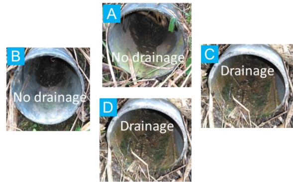
Figure 9 Drainage condition of drain pipes during prospecting
