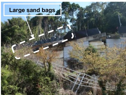
Figure 12 Placement of anti-weathering sand bags
