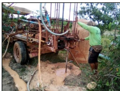
Figure 3 Water well being drilled for groundwater data
