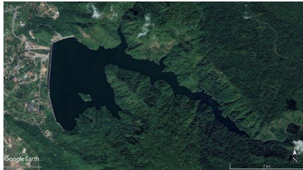
Figure 3 Khun Dan Prakan Chon Dam on 2 December 2019
