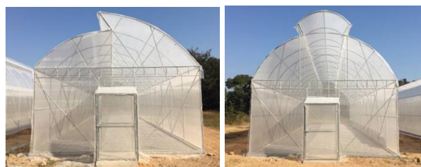
Figure 5 Prototype of Greenhouse with sawtooth and double roof.
