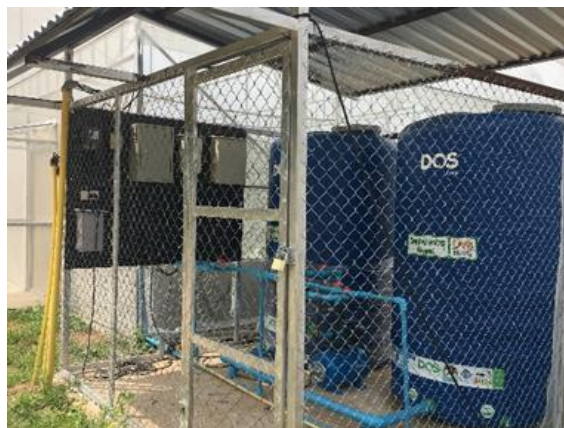
Figure 6 Installation of pumps and control systems, water supply in the Greenhouse.
