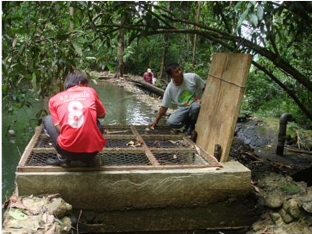
Figure 5.17 Sludge Filter was Installed in the Weir
