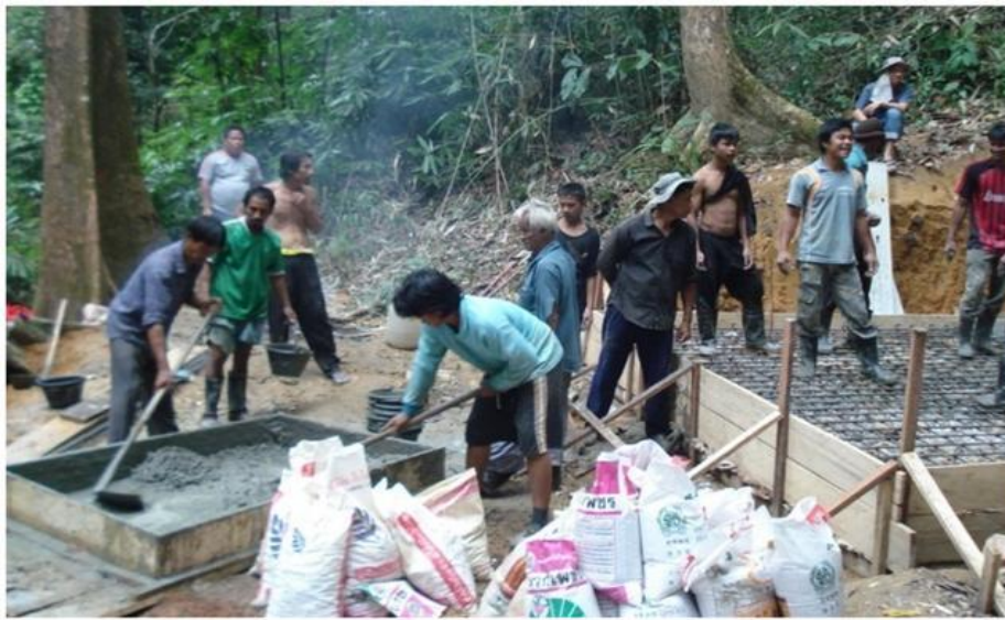
Figure 6.16 Reinforced Concrete Floor Construction Implemented by the Villagers
