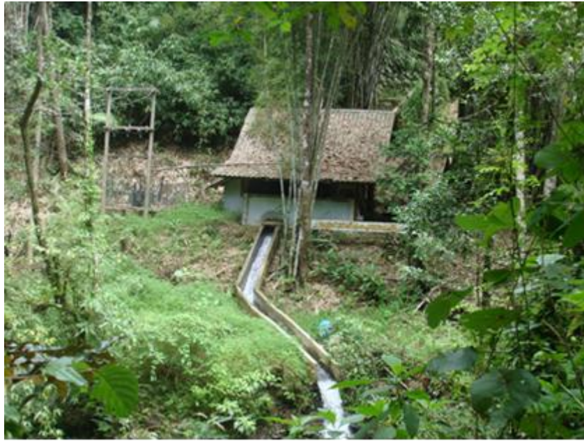
Figure 5.20 Drainage from Power Plant Building to Stream without Affecting Villagers
