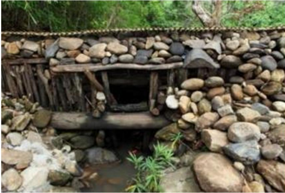
Figure 5.7 Natural Weir at Mae Pon Creek Constructed by Villagers
