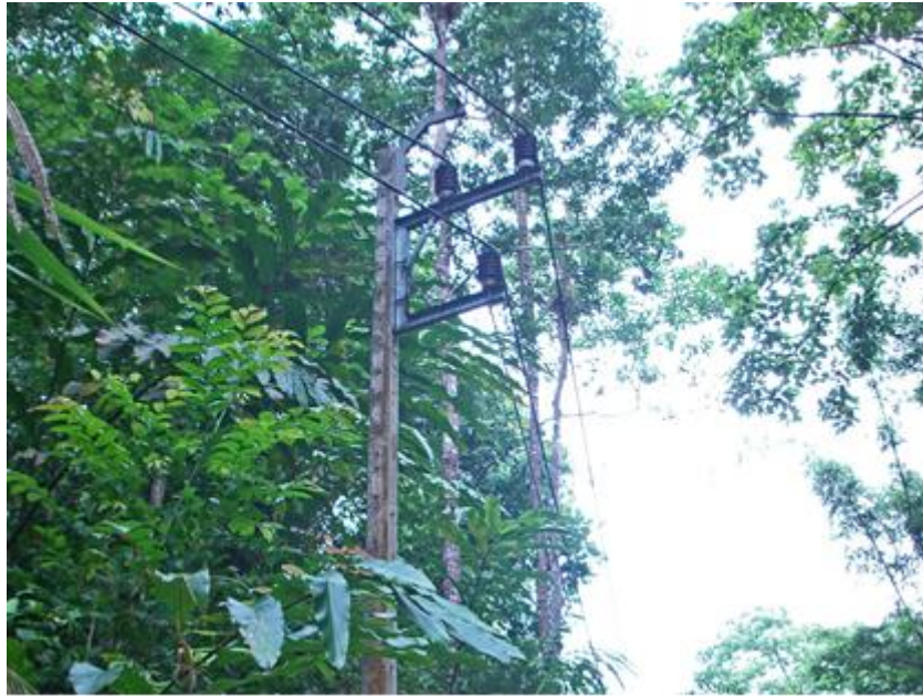
Figure 5.22 Transmission Line Installation Avoiding Big Trees
