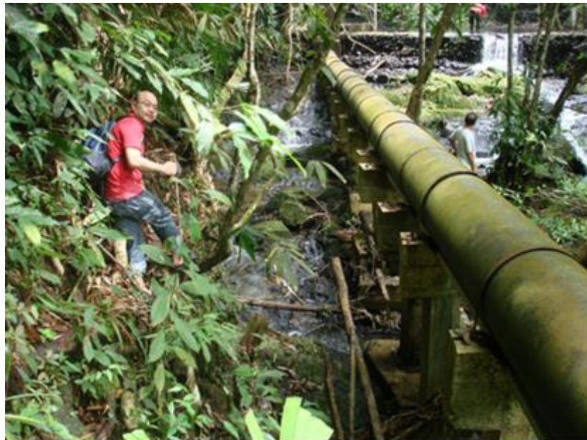
Figure 5.19 High-Pressure Polyethylene Pipeline Installation from Weir to Power Plant Building
