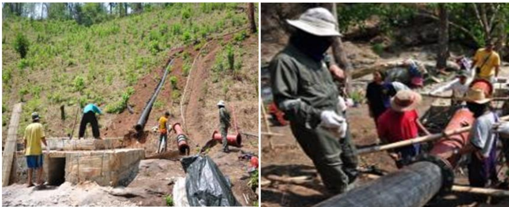
Figure 5.8 HDPE Pipeline Installation Carried out by Villagers
