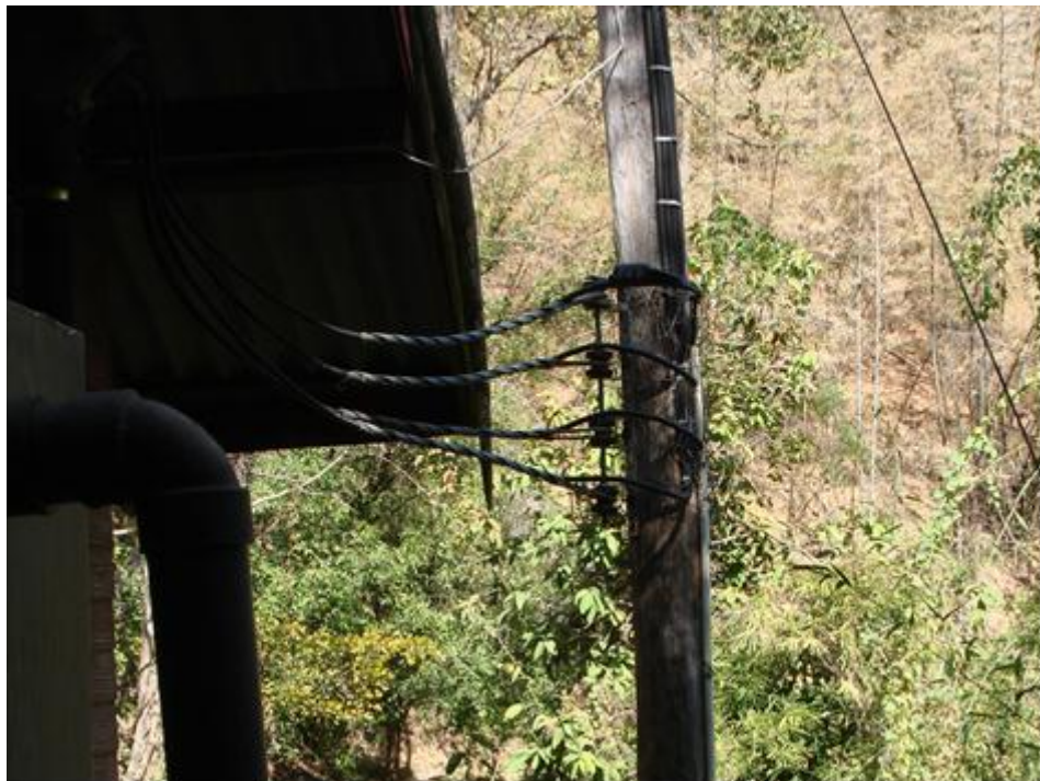
Figure 6.6 Transmission Line Attached to a Dead Tree
