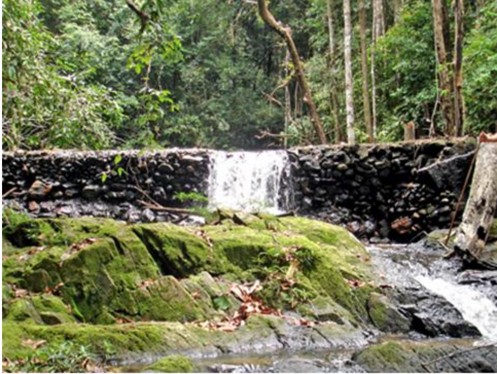
Figure 5.16 Weir Located Close to Haew Ta Jan Waterfall Constructed by Villagers
