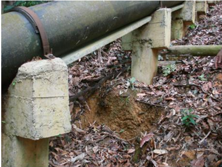
Figure 5.18 Construction of a Foundation for a High-Pressure Polyethylene Pipeline on Steep Slope
