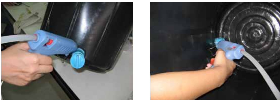
Appendix Figure A1 Drill the bucket and coat glue
