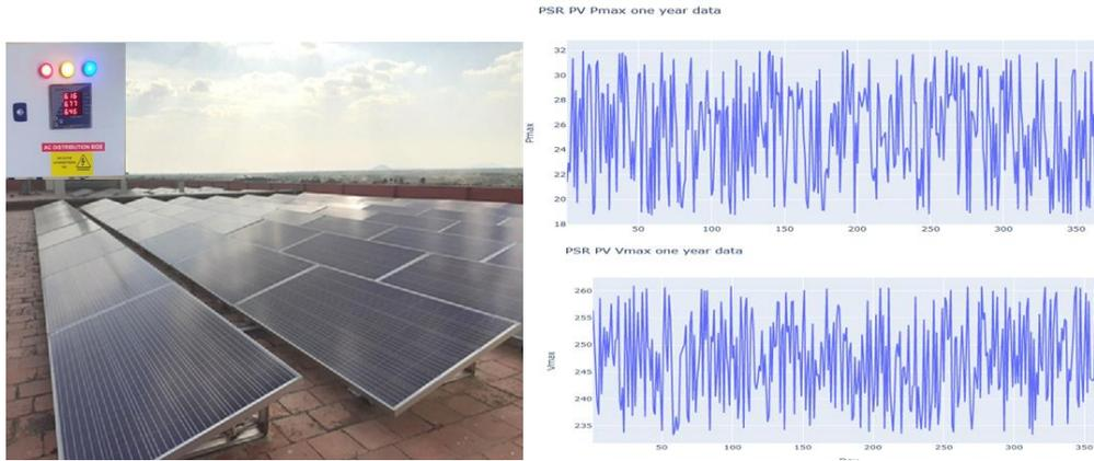
Figure 4. 33 kW real solar PV system, its data logger and Recorded value of  $P_{max}$  and  $V_{max}$  for 365 days
