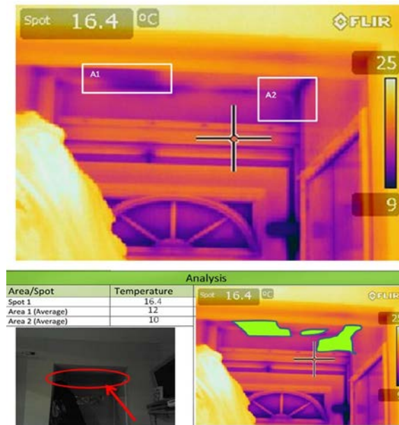
Figure 6: Using thermography for the entrance
