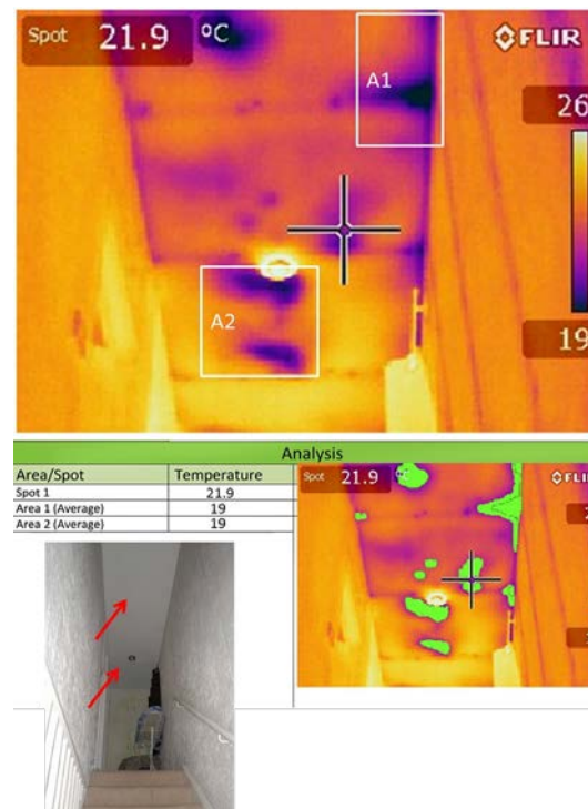
Figure 9: Using thermography for the staircase area
