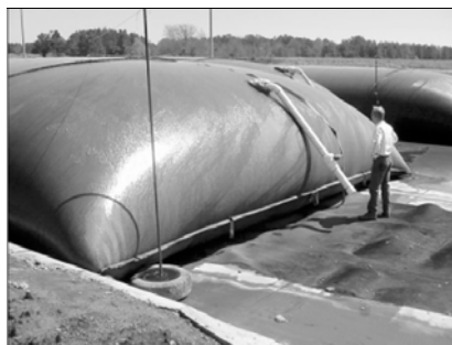
Figure 32 Schematic of Eco-tube method of reusing high water content soil. Source: Hirotoshi Mori and Hidetoshi Kohashi (2005)
