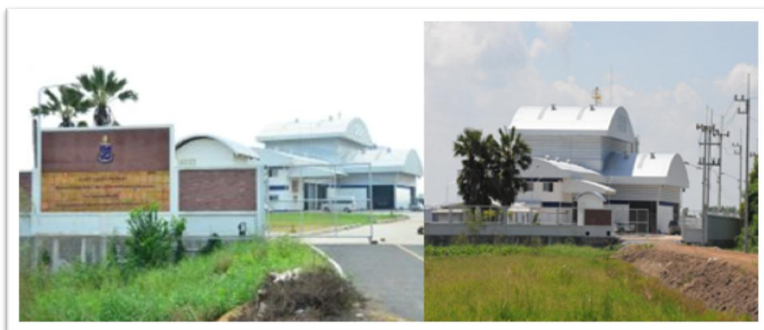
Figure 5.4 The Chaipattana Rice Mill (Demonstration and Integrated Renewable Energy Development and Demonstration Center), Lat Bua Luang District, Ayutthaya
