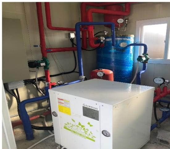
**Figure 2.** Geothermal heat pump system with heating tanks and water pipes.
