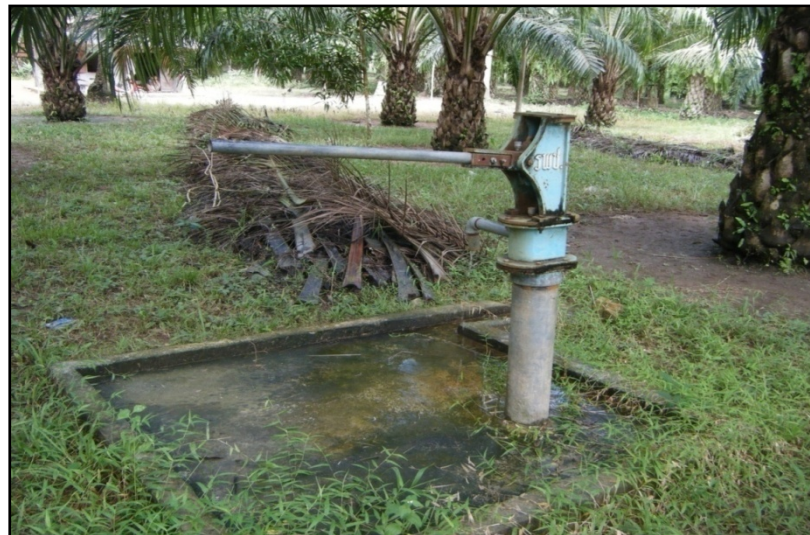
Figure 45 The second artesian well constructed by the Office of Accelerated Rural Development (ARD) in the middle of BTS.
