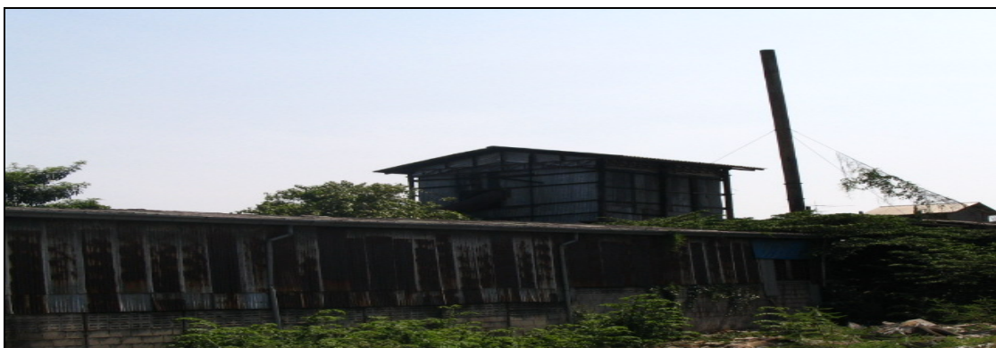
Figure 23 Foundry factories at present in Phetkasem 51 Road, Bangkhae
