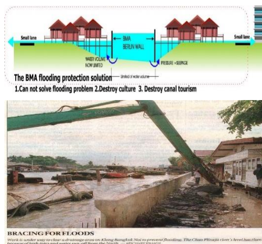
Figure 11: Sketch of BMA concrete wall cross section through canal and photo during construction (Authour).
