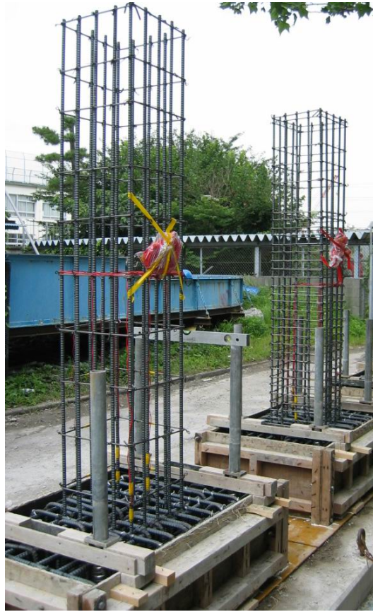
Appendix Figure 3 Reinforcement steel cages
