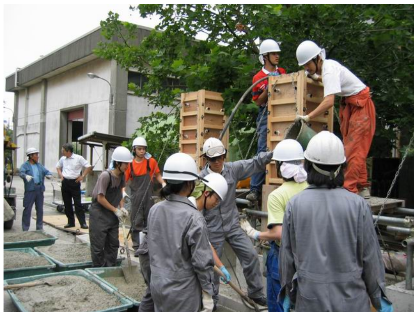
Appendix Figure 4 Concrete casting
