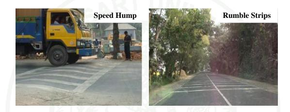
Figure 21 Speed reducing structures on N5
