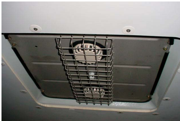
Figure 31 A Pair of Smoke Detector Installed
