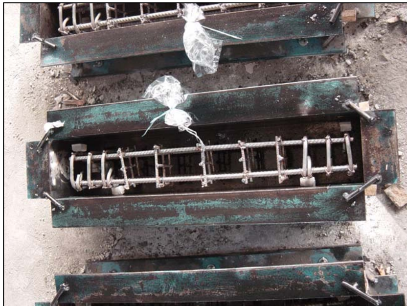
Appendix Figure D10 Preparation of formwork
