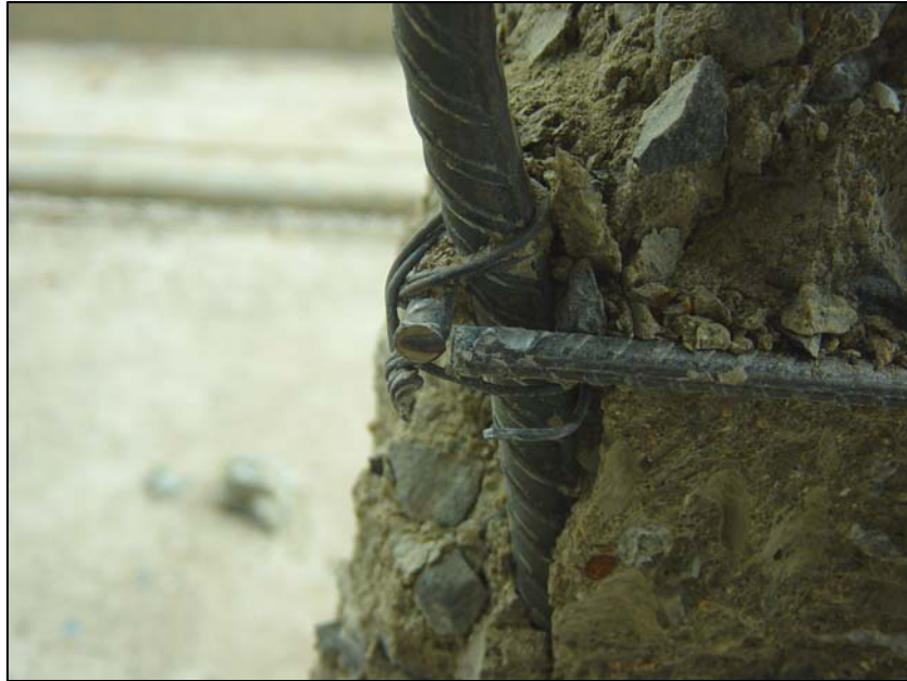
Figure 24 Failure of welded wire reinforcement (CDR6/2(10))
