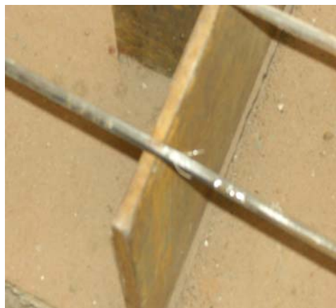
Figure 39 The joint at transferred plate to checkered plate welded for the first test in actual test.
