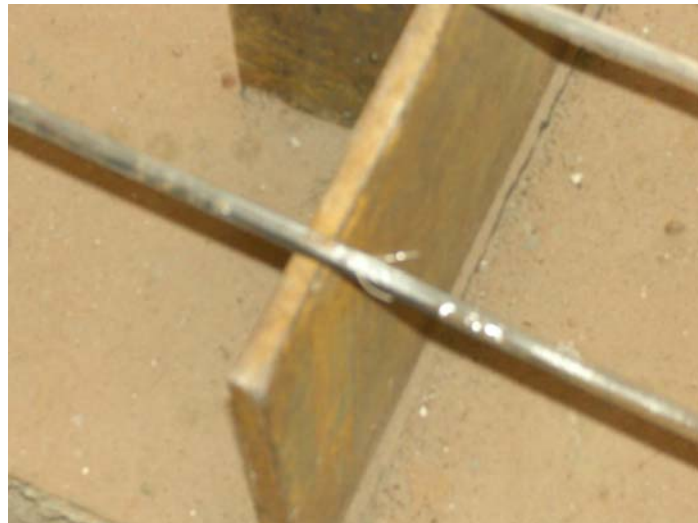
Appendix Figure C10 Strain gauges installed to the rebars
