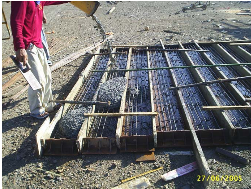
Appendix Figure C5 Concrete pouring
