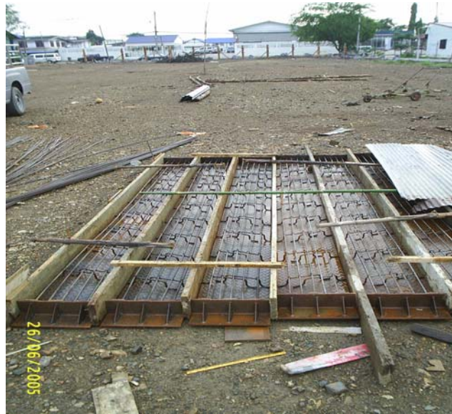
Appendix Figure C1 Reinforcement preparation
