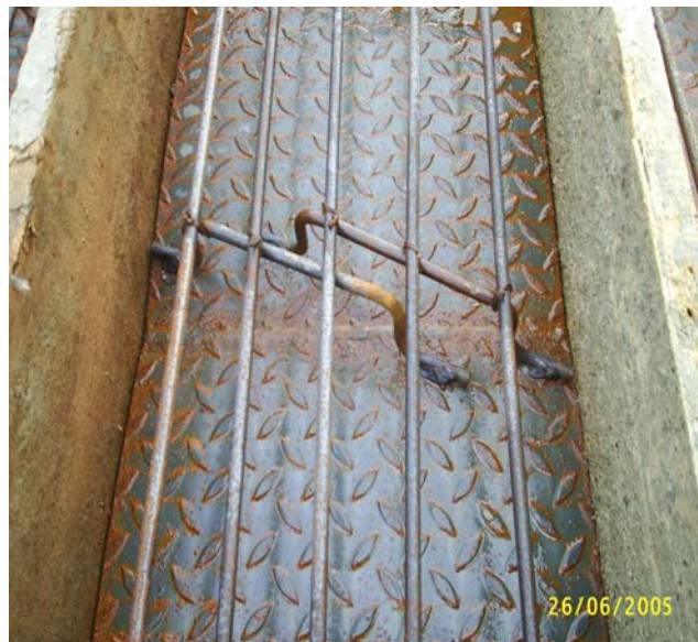
Appendix Figure C2 Shear key
