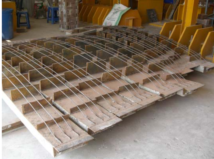
Appendix Figure C7 Transferred plates and rebars installed
