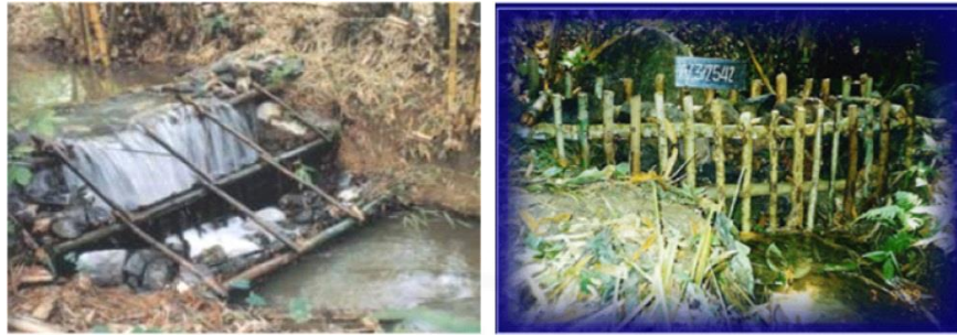
Figure 2-8 Local Weir (Combination Pattern)
