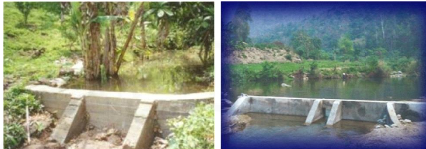
Figure 2-10 Check Dam with constructed by reinforced concrete (permanent)
