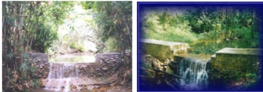
Figure 2-9 Check Dam with constructed by stone (Semi-permanent)
