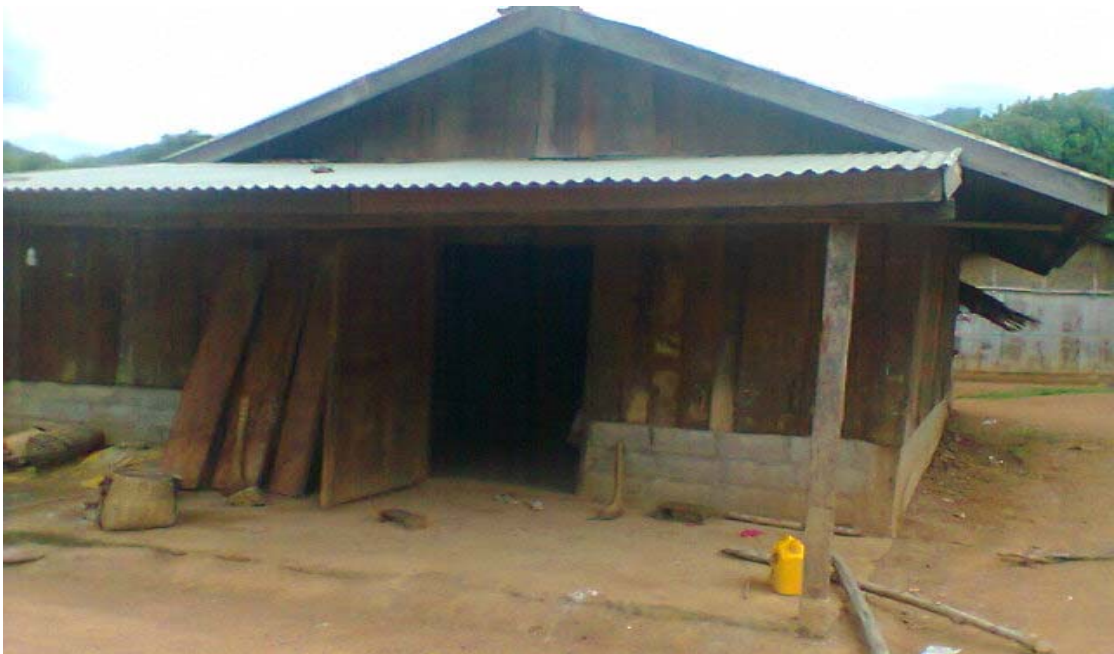
Figure 4.4 Style of new house made of wood, brick and magnate roof Photo by Phonesavane Sivily
