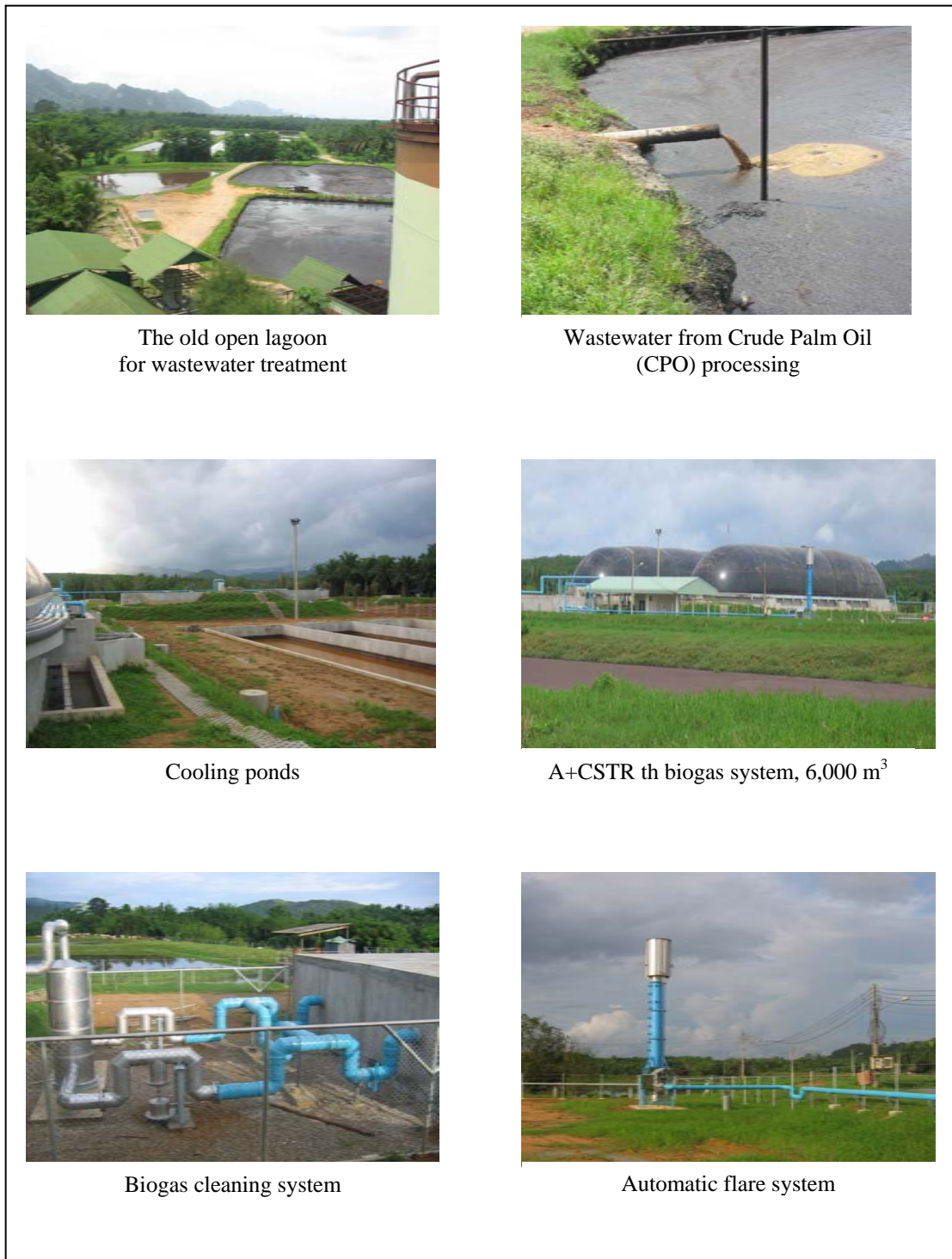
Figure 2-11 The implementation of biogas system in palm oil industry
