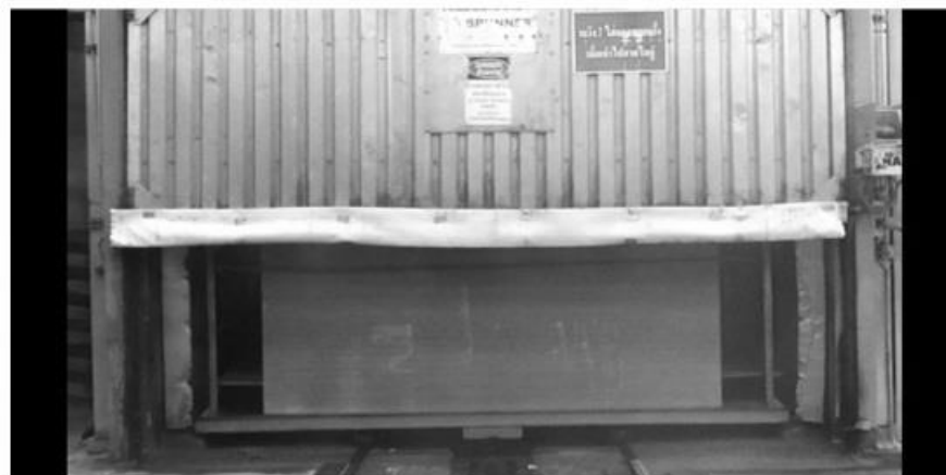
Figure 4.6 Hot air and steam released to the working space once the door opened
