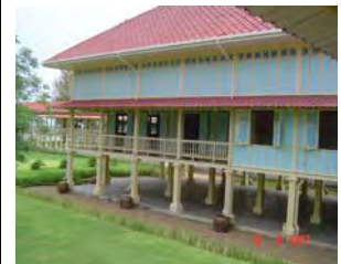
Figure 176 Openings for ventilation covered with framework (taken by Muangyai, N, 15/09/07) - The layout of the complex reminds the users of a large traditional Thai house with balconies walkways, and terraces.
