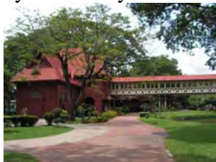
Figure 178 Marierajrattaballang Royal House and the covered walkway to Chaliemongkolasana Royal House (taken by Muangyai, N, 16/09/07)
