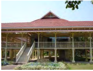
Figure 109 The staircase to residence of the Grand Chamberlain (taken by Muangyai, N, 29/01/09)
