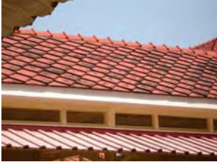
Figure 96 Rhombus-shaped roof tiles (taken by Muangyai, N, 29/01/09)
