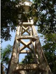
Figure 75 Water supply system (taken by Muangyai, N, 24/01/09)
